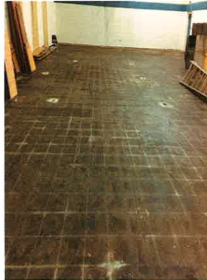
View showing ACM floor tiles removed in older north section of the school bldg.
