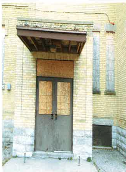
North West Entrance to the School Bldg.
