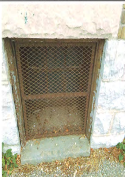
Wooden framed Basement windows. (Typ.) west side of Bldg.
