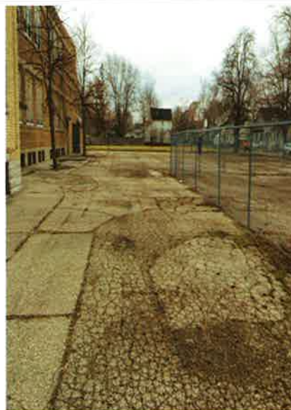
Asphalted Parking lot west of the School Bldg.
