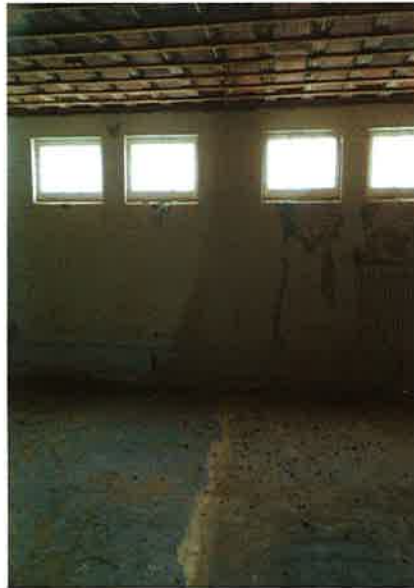
View showing ACM floor tile, and ceiling removed in older north section of the school bldg.
