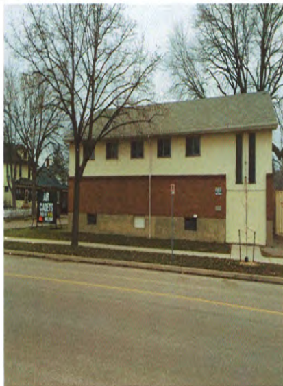
Looking north over Devine Street, to Air Cadets Bldg,
