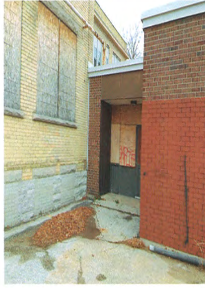
Looking north at view of Annex located at east of School Bldg.
