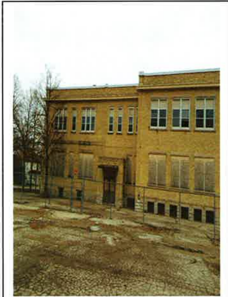
Looking north east, view of School Bldg.
