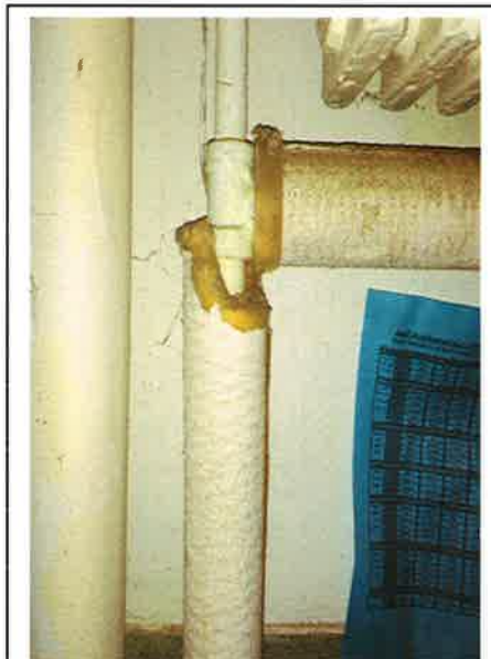
Non ACM insulation in Basement Utility Room
