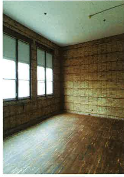
View showing ACM floor tile, wall and ceiling removed in older north section of the school bldg.
