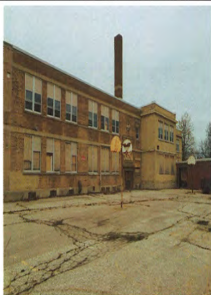
View of playground at the north east side of the Bldg.
