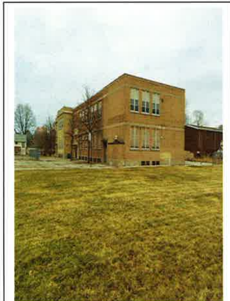
Looking north, view of School Bldg. and abutting adjacent field.
